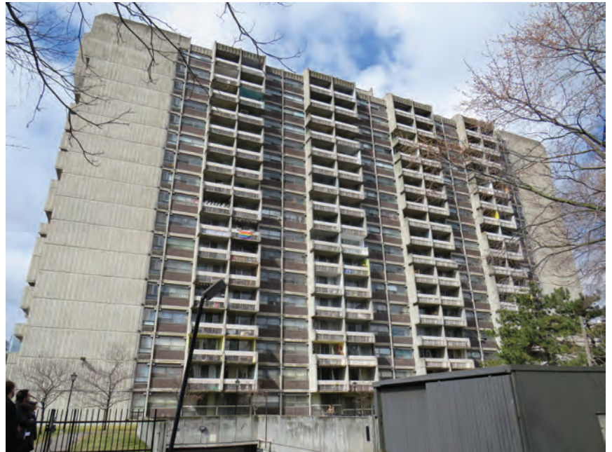
Fig. 2: Centrepont East South Building
